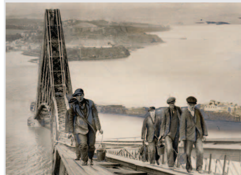
Painters walking up the Queensferry cantilever on the Forth Bridge in 1931. In the past, painting the Forth Bridge was highly labour intensive and especially treacherous. Painters would wear no gloves, no helmets, indeed no recognisable form of safety protection © Daily Mail
